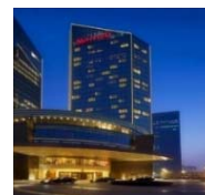
Beijing Marriott Hotel Northeast
