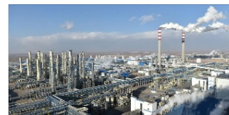
Shenhua Ningxia CTL Plant
